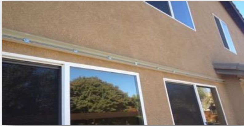
Wall attachment (Stucco application)
