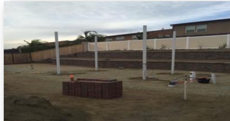
Free Standing (Steel Posts in concrete footings)
